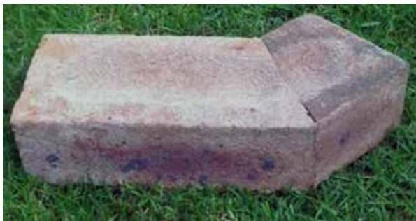
A Cut and Bonded External Angle
