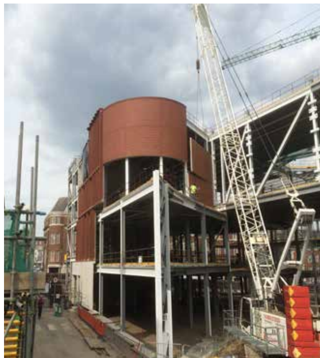
ACME Victoria Gate Arcade, Leeds.
