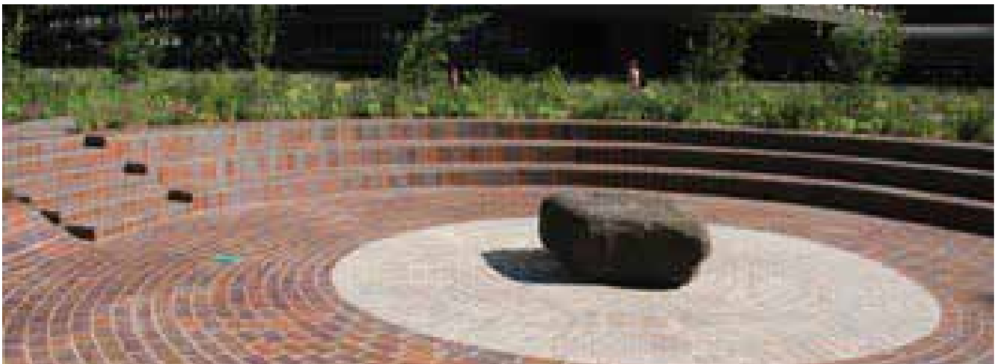
Rigid clay pavers at the Barbican, London ©
