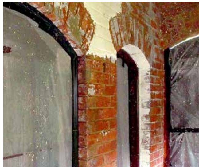
Further layers of paint may require an alternative treatment
