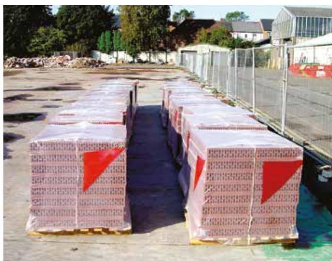
Stored bricks must be protected from inclement weather.
