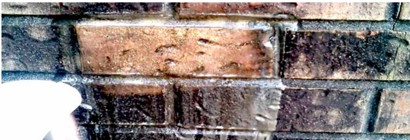
Detergent solution used to clean an internal fireplace
