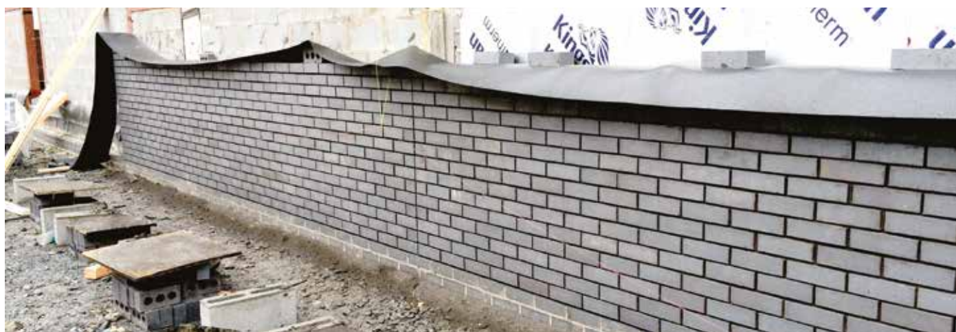
Bricks protected from rainfall, including stacks.
