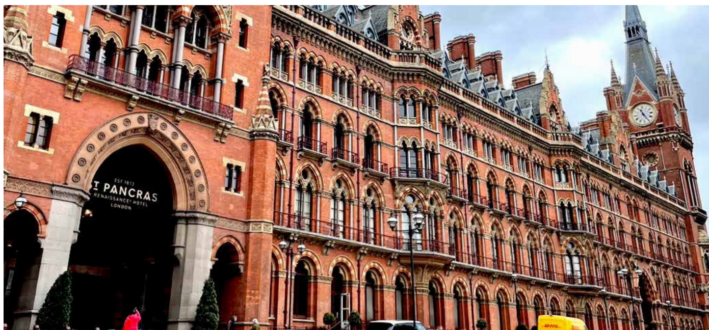
The result of cleaning brickwork can be spectacular.
