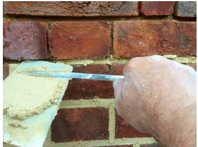
Repointing with lime mortar
