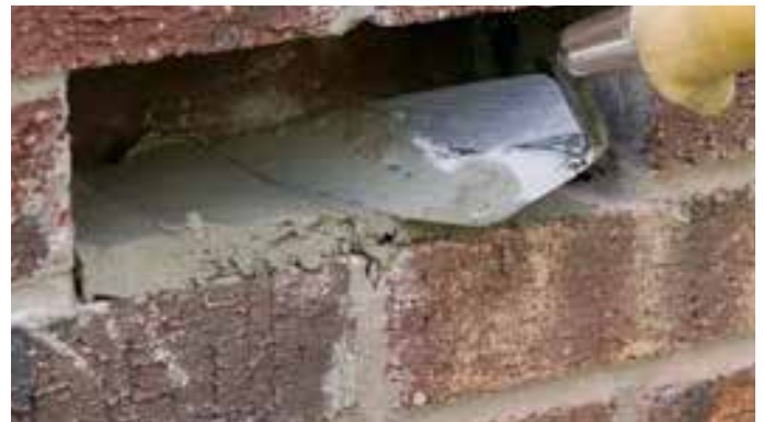
Apply mortar to three faces of brick and slide into place
