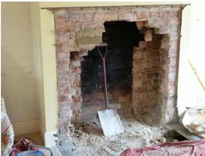
Careful assessment is needed prior to removal
