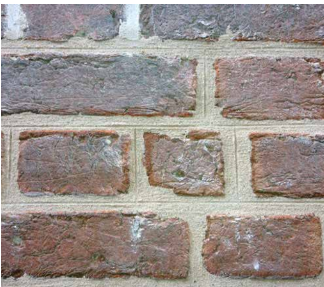
Jointed Flush Pointing
