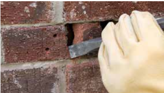
Cut out damaged brick
