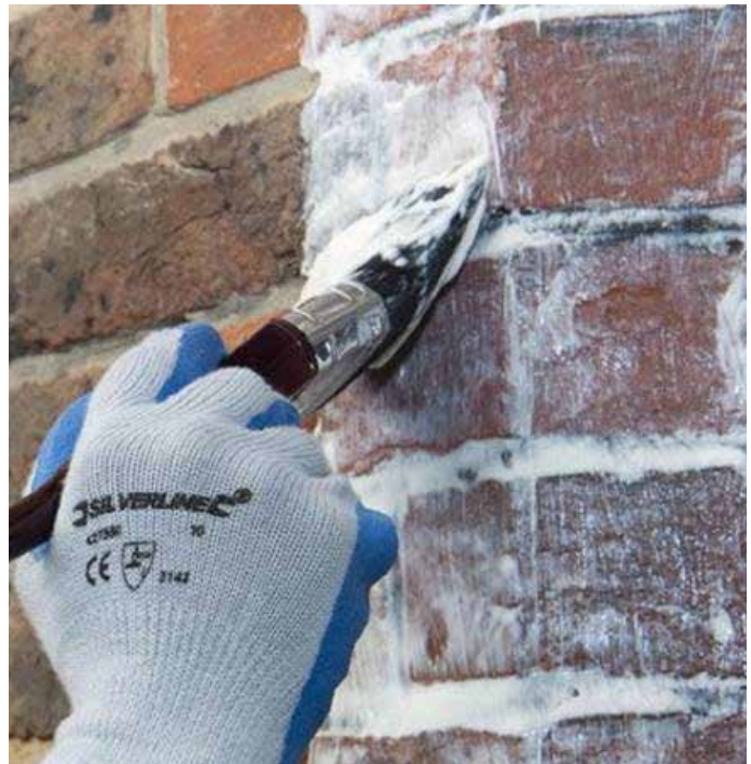
Masonry cream can reduce water penetration
