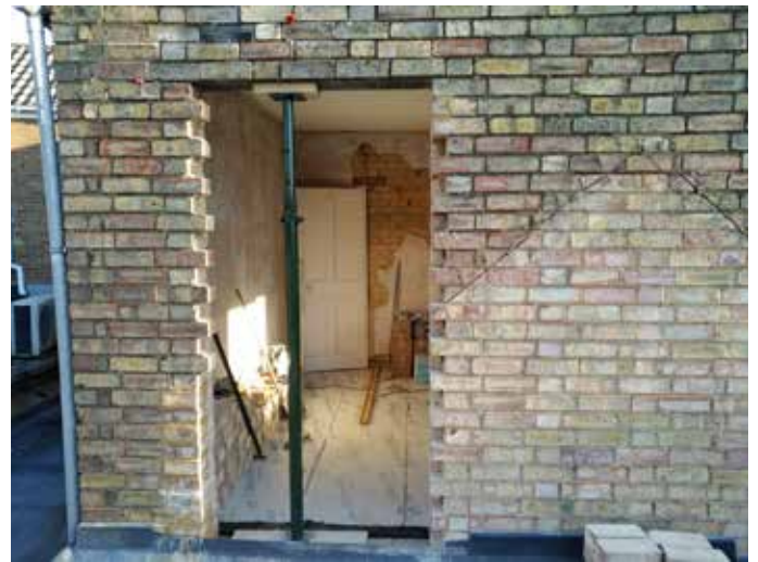
A new opening formed in an existing wall
