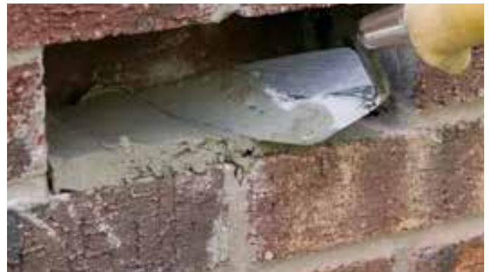
Apply layer of mortar to cavity bed
