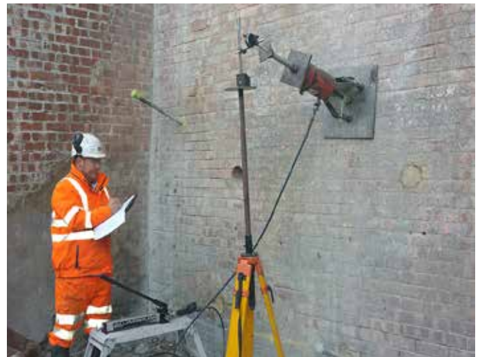
Structural tie installation for retaining wall
