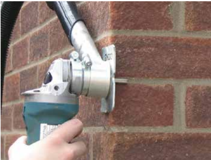
Raking out mortar joints
