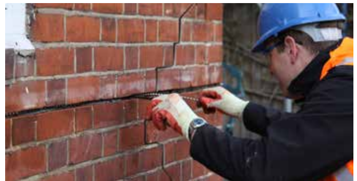
Helifix - insert reinforcement bar
