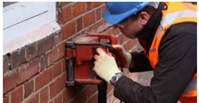
Helifix - cut out bed joint either side of crack
