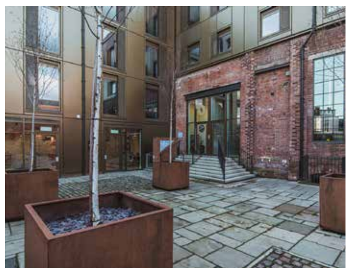
Thermal upgrades with bronze aluminium cladding.
