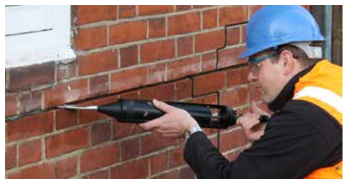
Helifix - inject the mortar and finish joint
