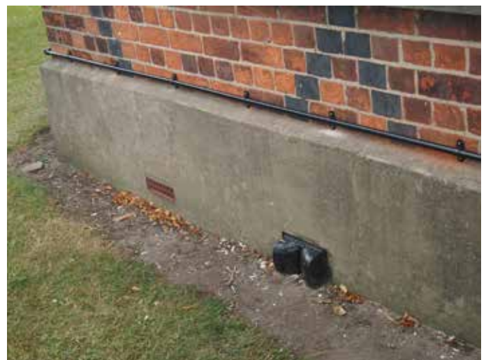
Concrete plinth to be removed
