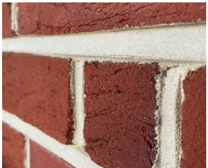
Weather Struck Jointing
