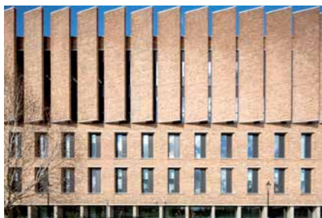
Precast panels to create details unachievable in hand set construction
