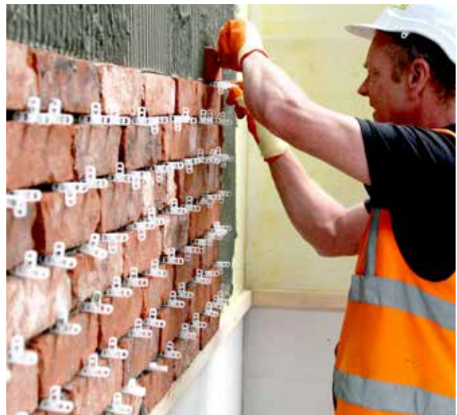
Brick slips used internally
