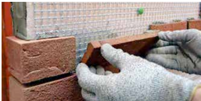
Mesh backing board to improve adhesion
