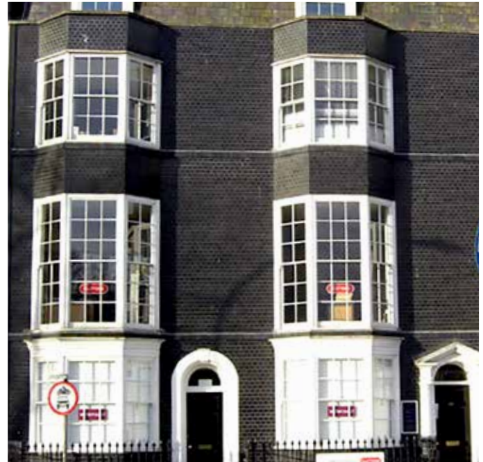
Timber framed property clad in mathematical tiles
