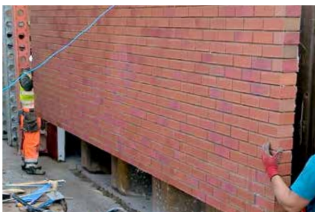
Single skin prefabricated brickwork
