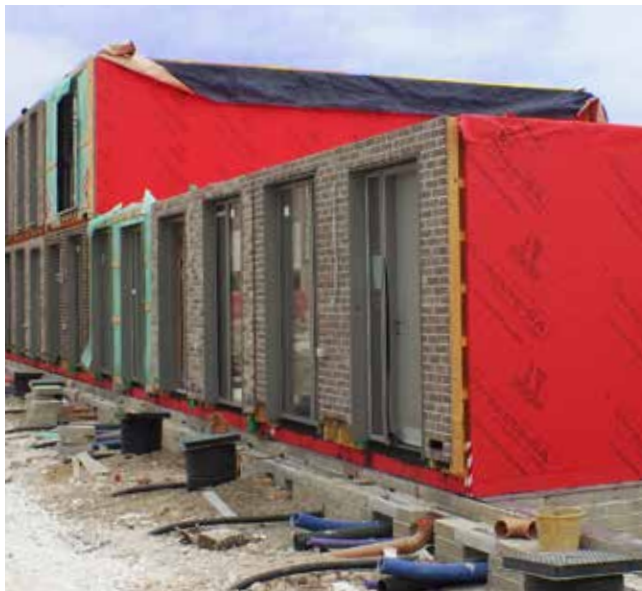
Panel system on 3D primary structure
