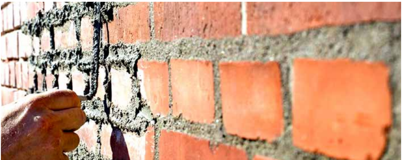
Efflorescence on brickwork under construction
