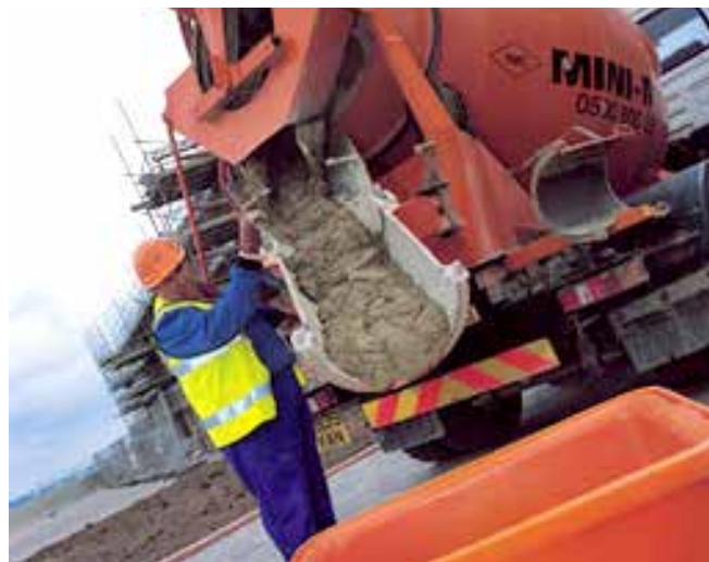
Mortar being delivered to site.
