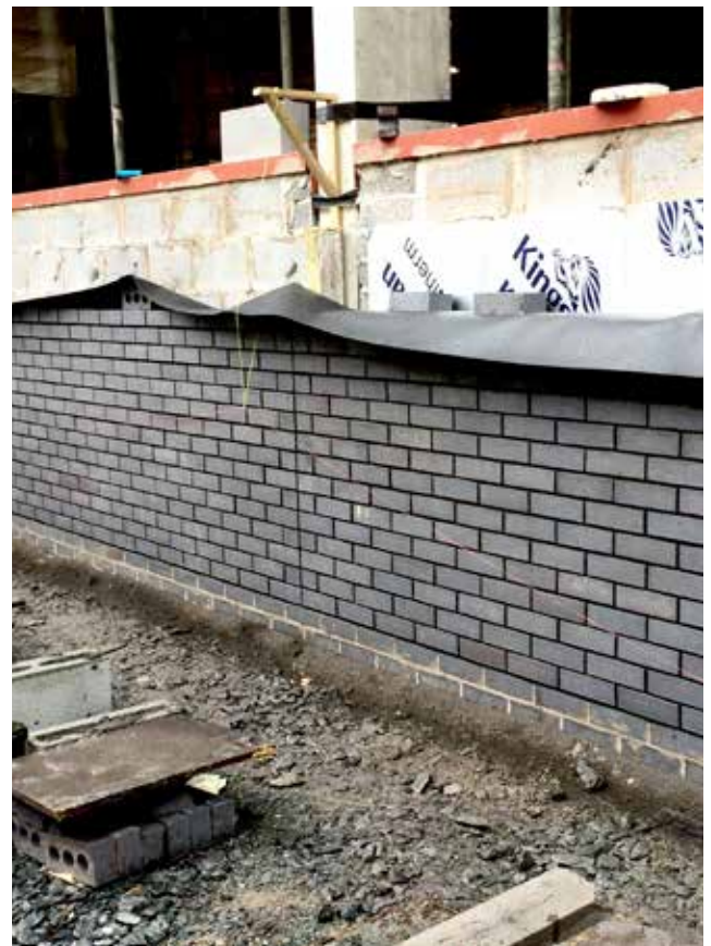
Protecting mortar from inclement weather is essential
