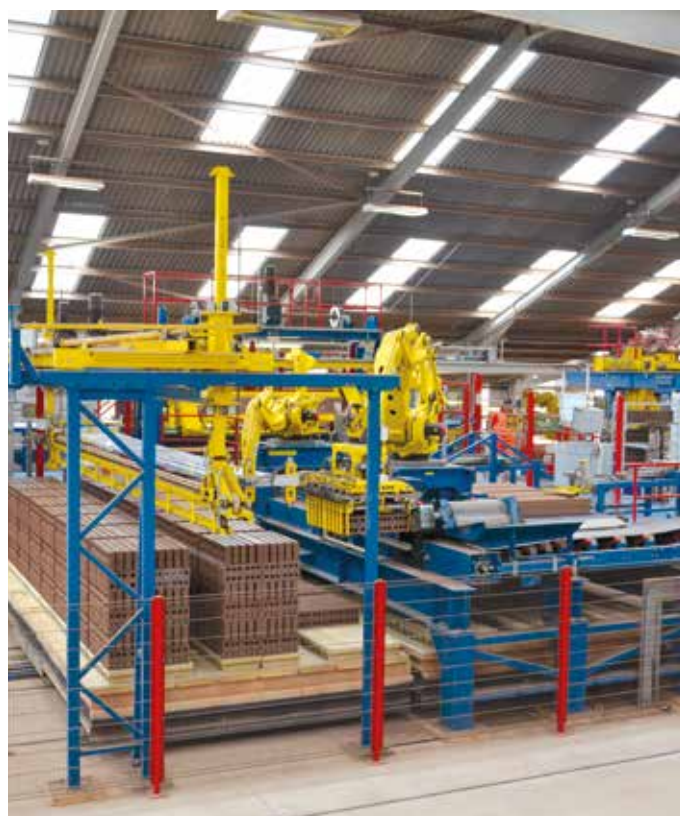
Kiln car drying
