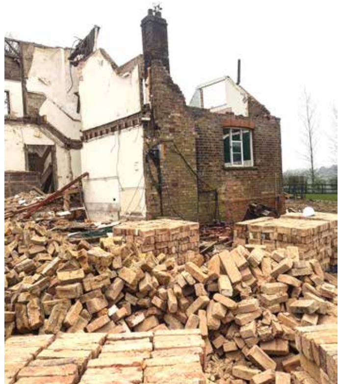
Stored bricks must be protected from inclement weather.
