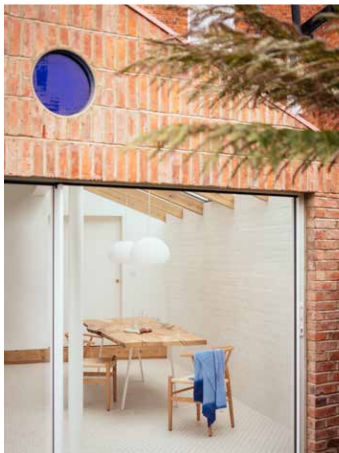
VATRAA; London Victorian house extension detail, using recycled bricks from the demolition of the building's original flank and rear walls.
