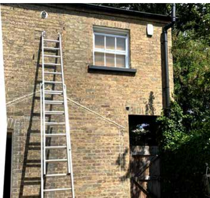
After applying solution to encourage lichens and mosses
