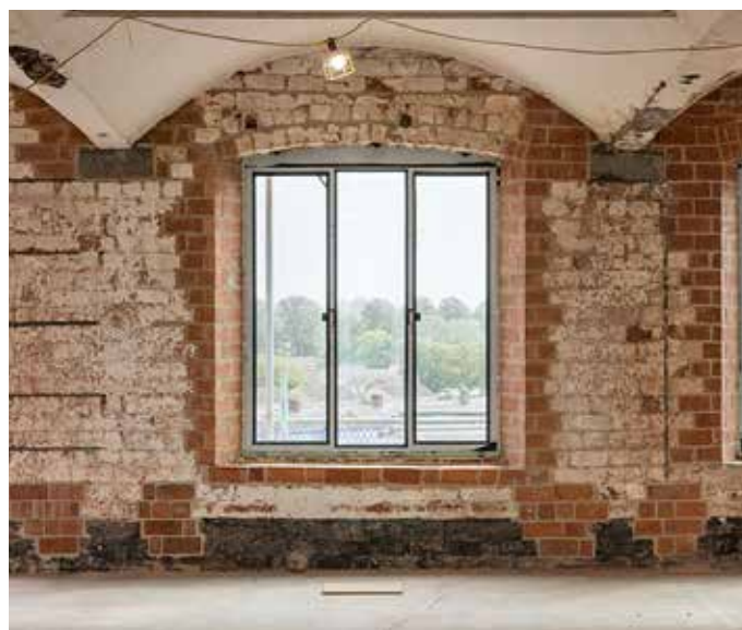
Historic England; Flaxmill Maltings Internal brickwork repair and replacement.
