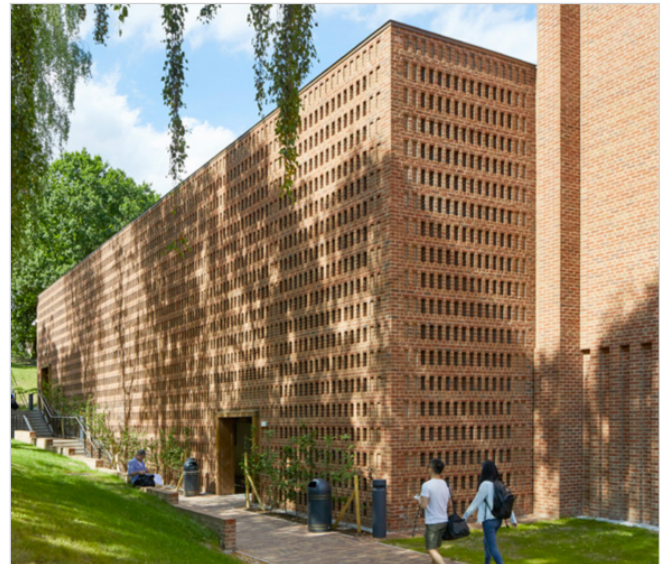
Hit and miss brickwork broken up in to smaller sections by the introduction of beams.
