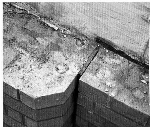
Figure 15a. Movement joint under construction.
