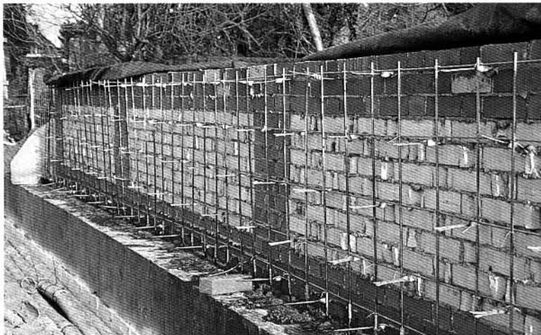
Figure 11. Reinforced brickwork grouted-cavity parapet wall under construction.
