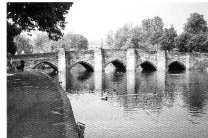
Figure 2d. Gothic arch.
