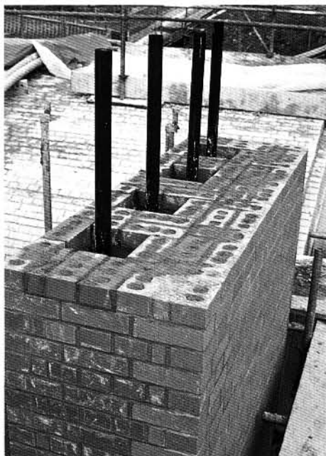
Figure 12. Post-tensioned walls.
