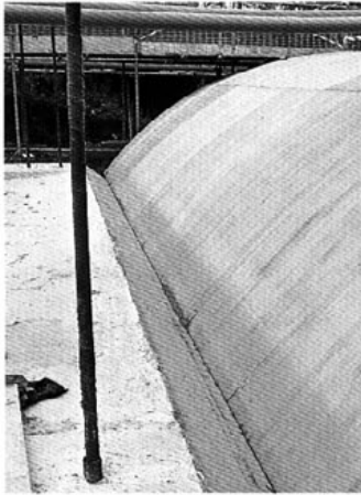
Figure 5. Foundation/springing.
