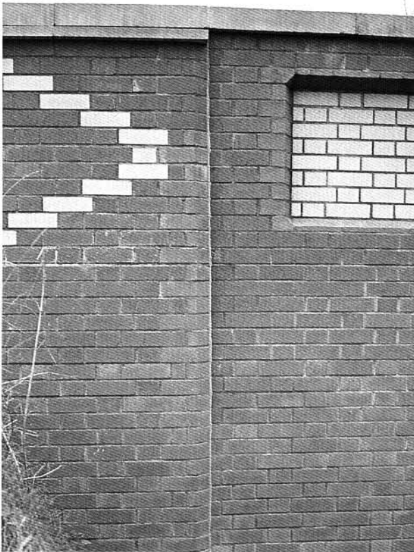
Figure 15b. Elevation on movement joint.
