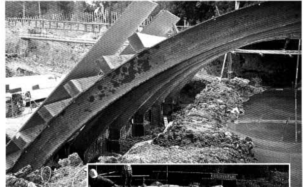
Figure 8. Kimbolton Centring. Inset: Brick arch barrel closing.
