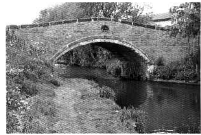
Figure 2b. Segmental arch.
