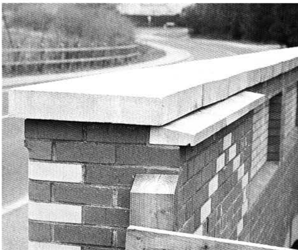
Figure 13. Copings to parapet walls.
