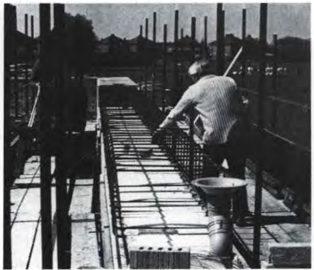
Above Reinforcement for an in situ capping beam. Sports hall, Ormskirk.
