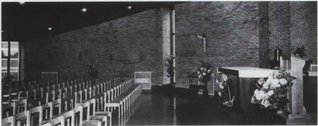
Above and right St Martin de Porres Church, Luton. Conflicting geometry of the walls and the roof created a structural problem. Making the walls and the roof structurally independent of each other, left the 7.7 m high walls surrounding the sanctuary standing as unpropped cantilevers and vulnerable to heavy wind loads. Diaphragm wall construction overcame this difficulty. Internally, full height windows set in the deep reveals of the diaphragm walls provide subdued yet dramatic natural lighting. Architects: Ellis Williams Partnership. Structural engineers: W. G. Curtin & Partners.
