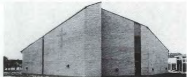
Above and right St Martin de Porres Church, Luton. Conflicting geometry of the walls and the roof created a structural problem. Making the walls and the roof structurally independent of each other, left the 7.7 m high walls surrounding the sanctuary standing as unpropped cantilevers and vulnerable to heavy wind loads. Diaphragm wall construction overcame this difficulty. Internally, full height windows set in the deep reveals of the diaphragm walls provide subdued yet dramatic natural lighting. Architects: Ellis Williams Partnership. Structural engineers: W. G. Curtin & Partners.
