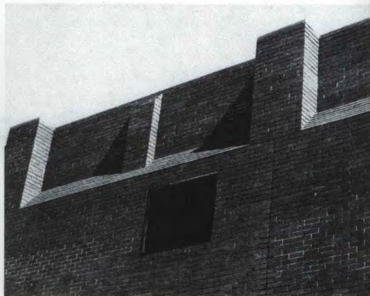
Top right and middle Swimming pool, Turton School, Bolton. Cross-ribs expressed externally. Architects: C. B. Pearson, Son & Partners. Structural engineers: W. G. Curtin & Partners.
