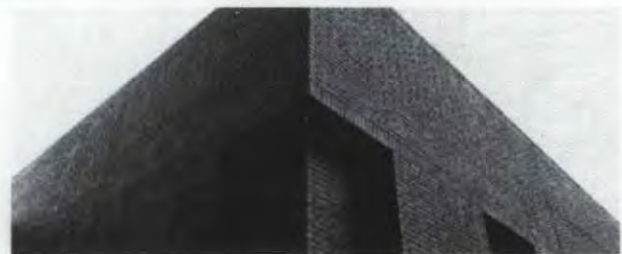
Below right Detail of workshop and stores building, Howley Park Brickworks, Dewsbury. Panels of conventional brickwork introduced at external corners provide visual interest and depth of modelling. Architect: S. E. Bell, DipArch RIBA (Head of Technical Services, George Armitage & Sons Ltd). Structural engineers: W. G. Curtin & Partners.
