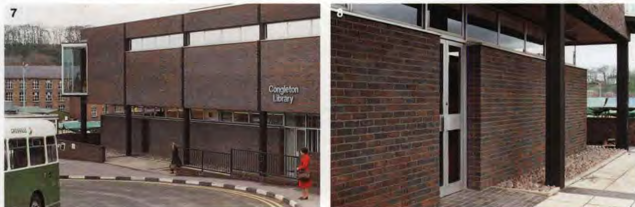
7 & 8. Congleton Library. Anxious to avoid an uninteresting rectangular box structure, the designers required the ground floor brick walls to be set back, well inside the perimeter frame. As clerestorey lights were required at this level, the walls are unrestrained cantilevers and, therefore, post-tensioned to resist wind loads. The first floor brickwork is not post-tensioned, being treated as panels spanning between rc columns. Architect: Cheshire County Architects Department. Consulting engineer: Curtins
