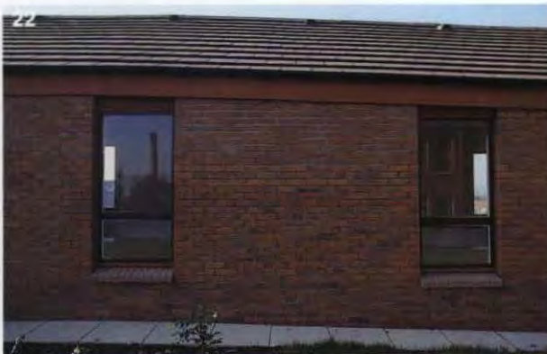
21, 22 & 23. Bolton District General Hospital. The link corridor was designed to have maximum natural lighting with full height windows, and to be constructed in brickwork, to match the predominant cladding/structural material throughout the hospital. The brick piers between the windows of the link corridor were post-tensioned, in order to carry the lateral window-loading which is very prominent in this location. The post-tensioned piers act as free cantilevers, as the pitched tiled roof structure is not capable of transferring load to any suitable shear walls or the like. Architect: Gilling Dodd Partnership. Consulting engineer: Curtins
