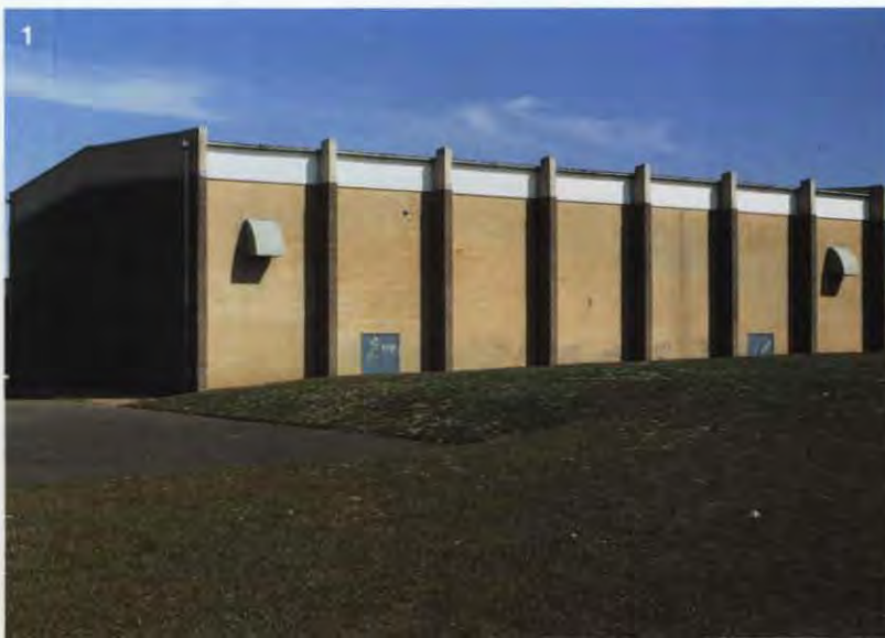
1 & 2. An early post-tensioned project, dating from 1967, by the authors. Several schemes were costed using steel frames and brick cladding. It was found that post-tensioned brickwork for the 10m high piers provided a more economical solution. Seeking a better solution for problems of the Flint High School Sports Hall, the diaphragm wall concept went on to develop into the fin wall. Later, the enormous potential of the post-tensioned diaphragm and the post-tensioned fin wall was recognised. Architect: Clwyd County Architects Department. Consulting engineer: Curtins
