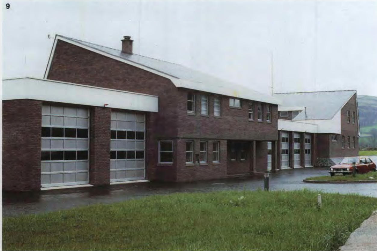
9. Corwen Emergency Services Centre. The architects wanted brick cladding to the slender columns between garage doors, and also wanted to avoid internal projections. Post-tensioned cavity brickwork provided a functionally superior and a much simpler and cheaper alternative to the more obvious choice of steel or rc columns. Architect: Clwyd County Architects Dept. Consulting engineer: Curtins
