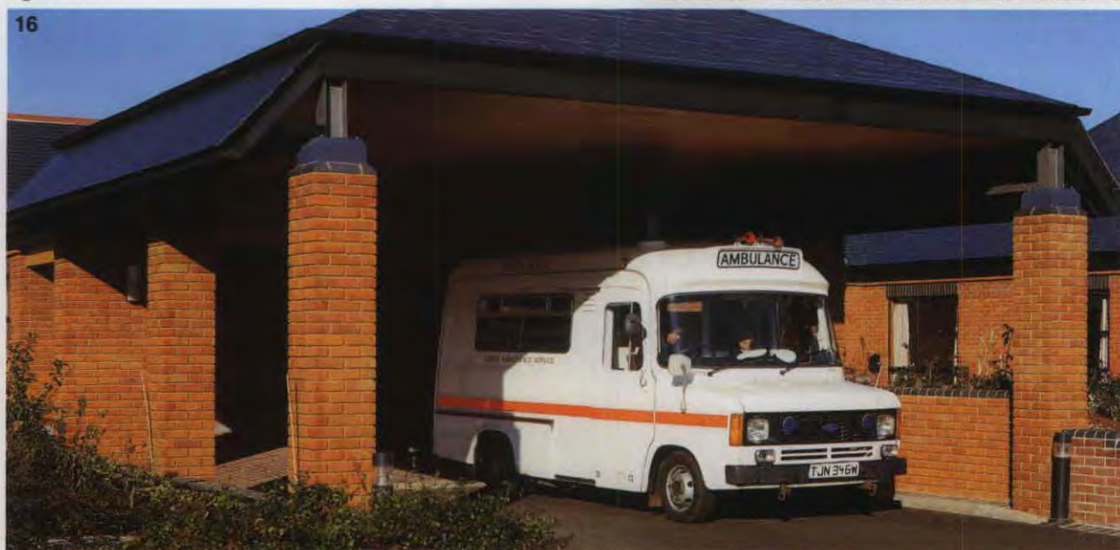
15 & 16. Ambulance Canopy, St Michael's Hospital, Braintree. The ambulance port forms the main entrance into the Rehabilitation Department, for both ambulances and the general public. Consequently, it was important to achieve an aesthetically pleasing appearance, whilst maintaining the overall purpose of providing shelter to incoming patients, during transfer between the ambulance and the hospital. The architect elected to use a tiled roof canopy on brick piers, without interconnecting side walls, to give an open structure on all four sides. Structurally, therefore, the problems were of overall long-term stability, and short-term stability after accidental damage due to impact. The supporting brick piers are a hollow-box, 440mm square, with a central void of 235mm through which two high yield 16mm diameter bars pass to post-tension each pier. The moment of resistance of each pier was thus increased by a factor of well over 8 times compared to a 440mm square solid brick pier, and its impact resistance was massively increased. Should a pier be accidentally removed, the post-tensioning rods also act as ties in the opposite corner pier, to prevent total roof collapse. Regional Architect: North East Thames Health Authority. Consulting engineer: Curtins
