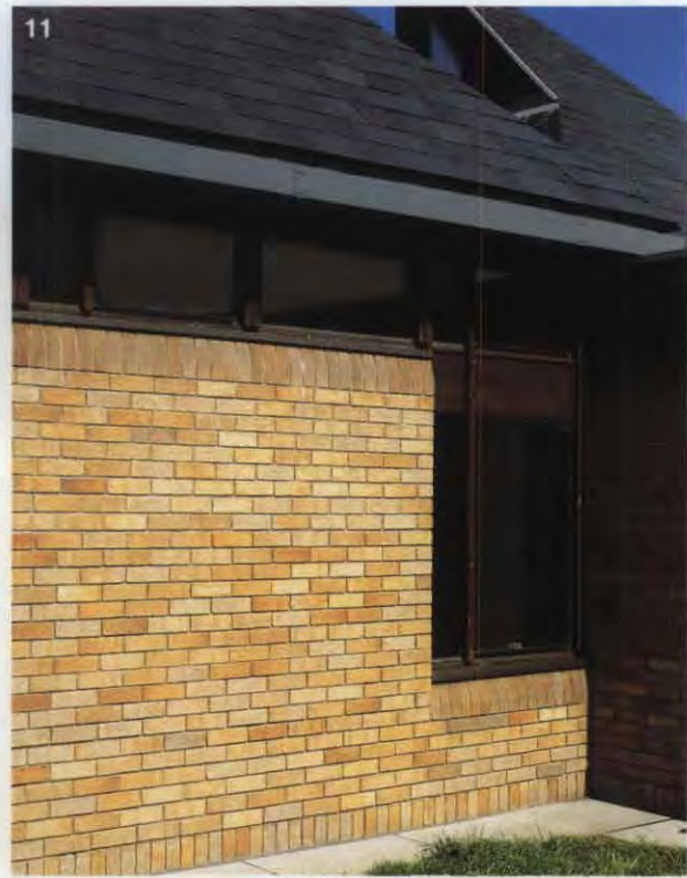
10 & 11. Rhyl Parish Centre. The roof is supported by a common steel column, at the central point of intersection, and by steel columns located at the corners of the four units. Bearing in mind its use as a church, clerestorey lighting was felt to be a functionally appropriate solution to the problem of providing natural light. Which meant, of course, that the perimeter walls would become unrestrained cantilevers and vulnerable to wind loads. Post-tensioning provided the answer. Architect: Weightman & Bullen. Consulting engineer: Curtins
