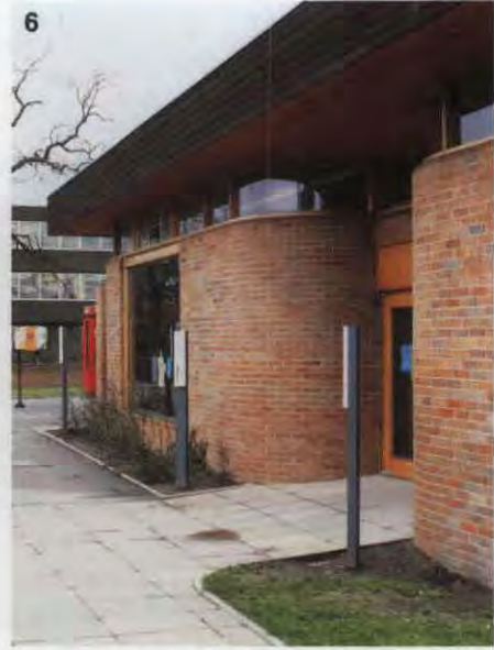
5 & 6. Barnnton Library & Handforth Library. These projects demonstrate another option of the SCD system. Both have a steel frame set well inside the building, with the roof cantilevered out. Using post-tensioned brickwork, one is freed from the restraints of the perimeter frame. In both these projects, the fenestration is precisely geared to the needs of the internal layout. Architect: Cheshire County Architects Department. Consulting engineer: Curtins
