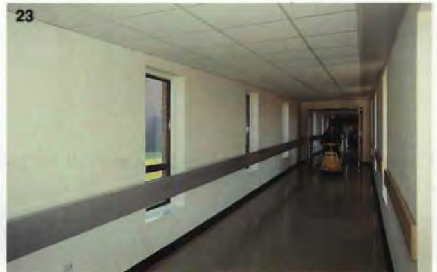
21, 22 & 23. Bolton District General Hospital. The link corridor was designed to have maximum natural lighting with full height windows, and to be constructed in brickwork, to match the predominant cladding/structural material throughout the hospital. The brick piers between the windows of the link corridor were post-tensioned, in order to carry the lateral window-loading which is very prominent in this location. The post-tensioned piers act as free cantilevers, as the pitched tiled roof structure is not capable of transferring load to any suitable shear walls or the like. Architect: Gilling Dodd Partnership. Consulting engineer: Curtins
