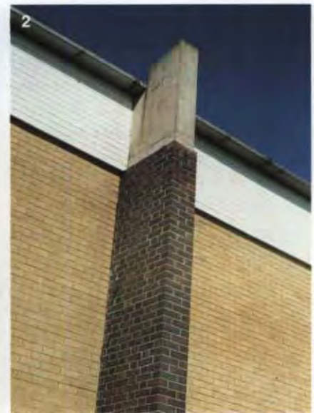
1 & 2. An early post-tensioned project, dating from 1967, by the authors. Several schemes were costed using steel frames and brick cladding. It was found that post-tensioned brickwork for the 10m high piers provided a more economical solution. Seeking a better solution for problems of the Flint High School Sports Hall, the diaphragm wall concept went on to develop into the fin wall. Later, the enormous potential of the post-tensioned diaphragm and the post-tensioned fin wall was recognised. Architect: Clwyd County Architects Department. Consulting engineer: Curtins
