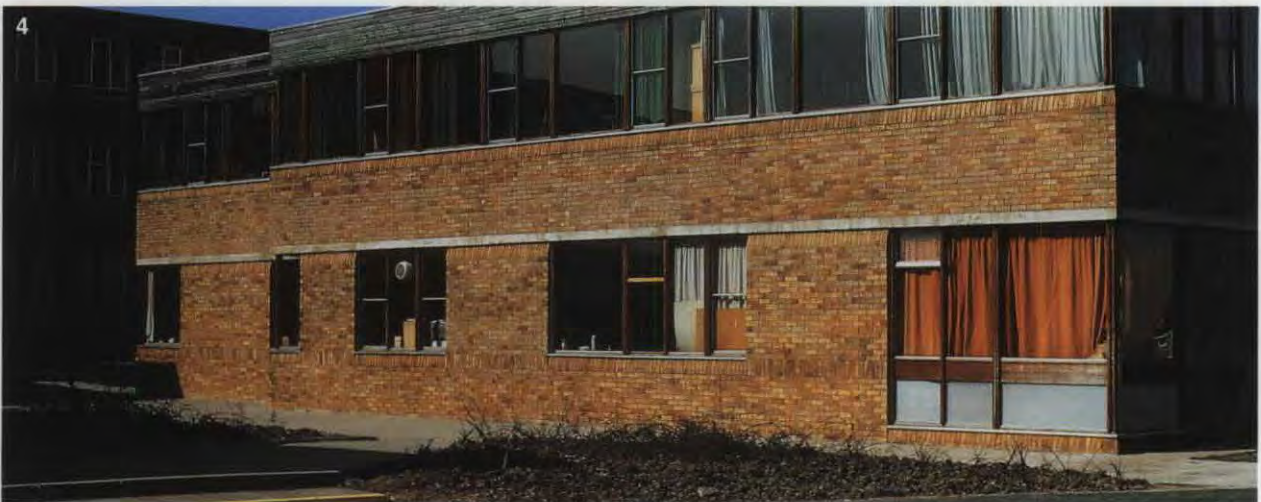
3 & 4. Studies were carried out to evolve a standard form of construction for Cheshire County Architects Department. The key element in the resulting SCD system is the post-tensioned brick cantilever wall. Holywell RC Primary School (3) is a good example of the varying brick panel heights and configurations with differing post-tensioning requirements. At Richard Gwyn High School (4) the first-floor brick spandrel walls, with the long runs of glazing over, are post-tensioned to the first-floor slab. Architect: Weightman & Bullen. Consulting engineer: Curtins
