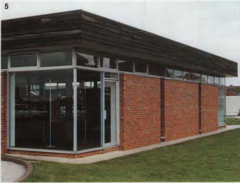
5 & 6. Barnnton Library & Handforth Library. These projects demonstrate another option of the SCD system. Both have a steel frame set well inside the building, with the roof cantilevered out. Using post-tensioned brickwork, one is freed from the restraints of the perimeter frame. In both these projects, the fenestration is precisely geared to the needs of the internal layout. Architect: Cheshire County Architects Department. Consulting engineer: Curtins
